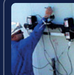
LARGE STRUCTURE INSPECTION (LSI™)
